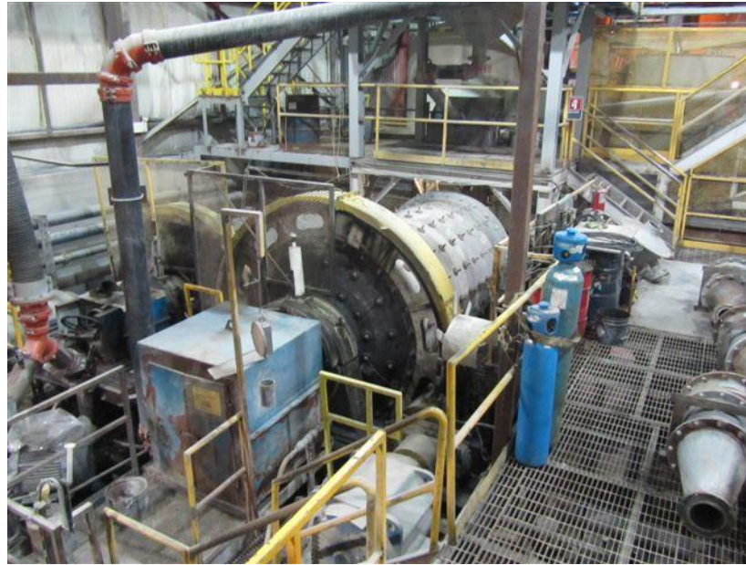
Figure 14: New Equipment Commissioned at Bachelor Mill
