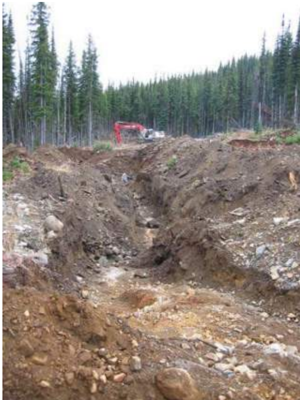
Photo #1b View looking South along Eagle Vein
